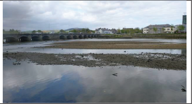
Plate 10: Gravel banks just downstream of bridge
